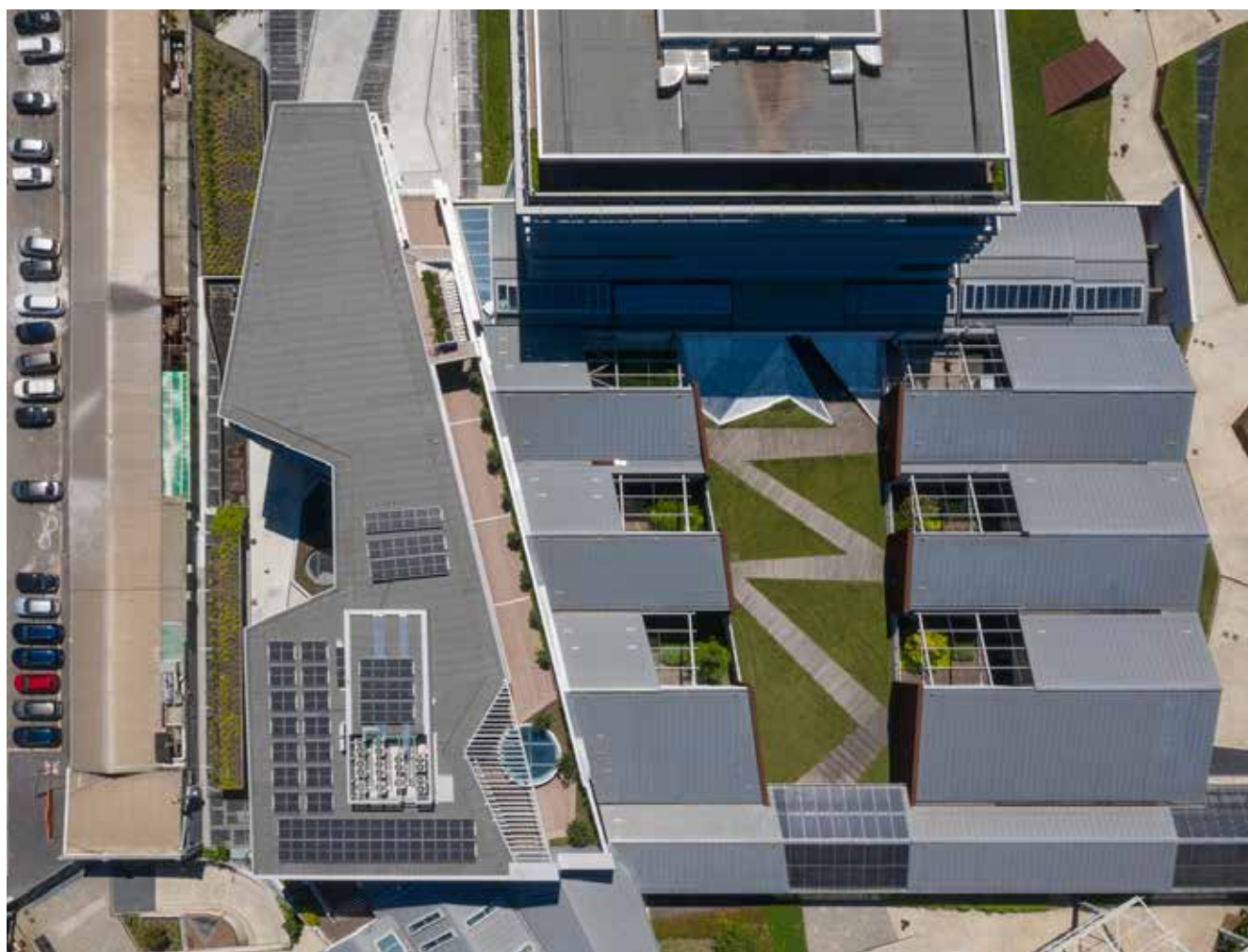
Top view of the new building designed by architect Giuseppe Tortato
